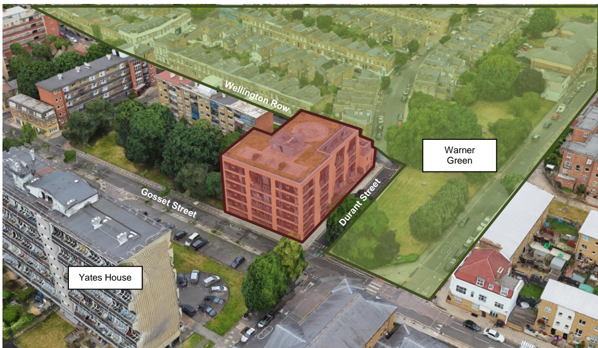
Figure 1: Site and surrounds. Site is highlighted in red. Jesus Hospital Estate Conservation Area highlighted in green.
