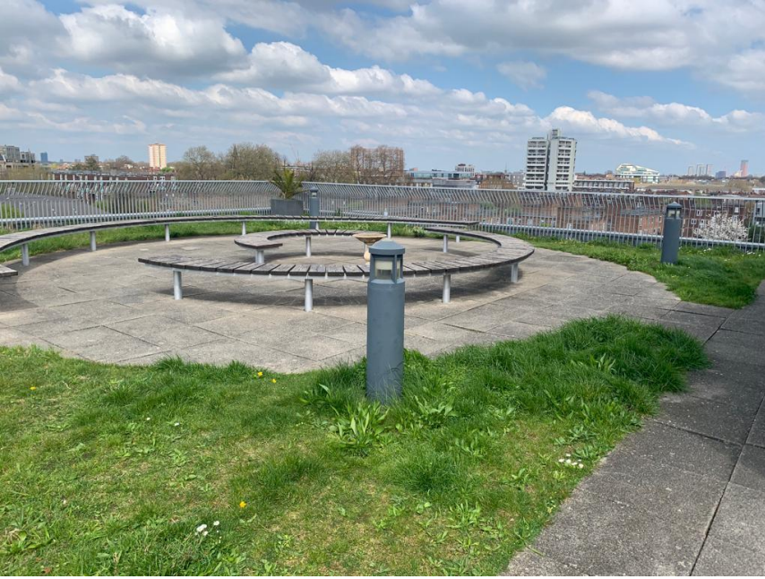
Southern section of existing roof garden
